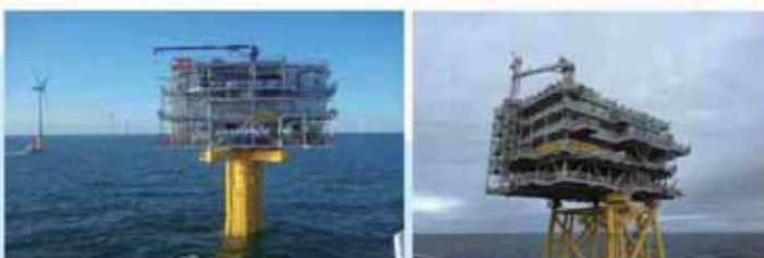
Figure 2/ Monopile Foundation and Jacket Foundation
