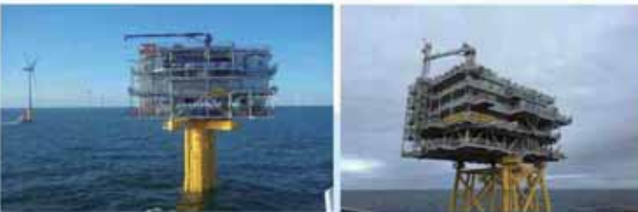
Figure 2/ Monopile Foundation and Jacket Foundation Source/ [4]
